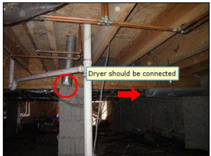
Dryer not connected
